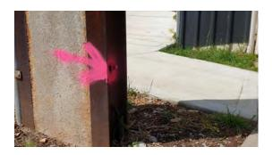
TBMs on a survey plan are depicted by a broad arrow. Whenever a TBM is established and a plan produced, some information regarding that TBM; a description of its location, how it can be identified, and the height of the TBM as it relates to the datum of the plan.
